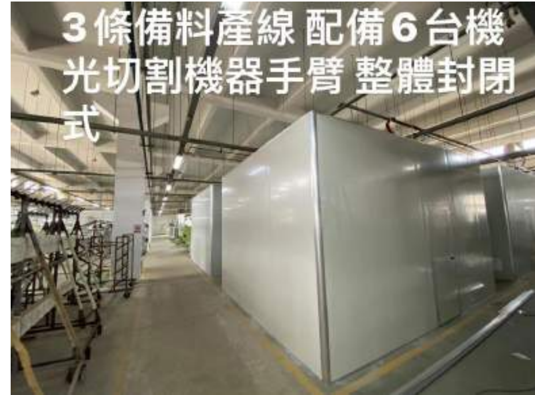
◆ 3 lines of material preparation with 6 laser cutting robots.
